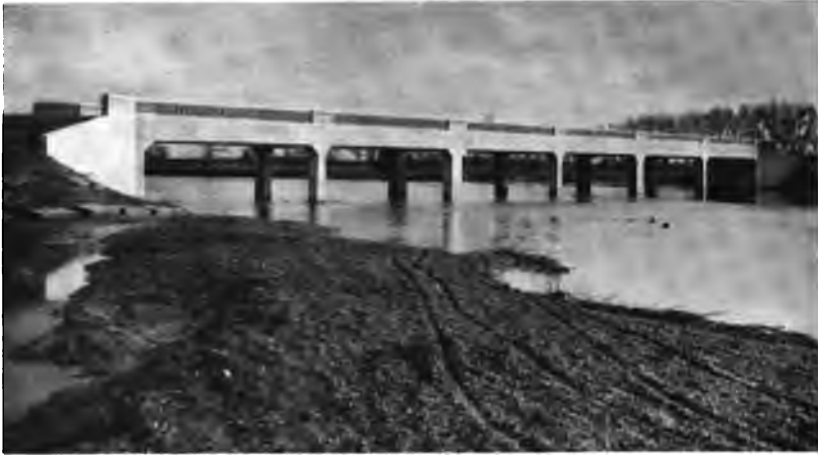
Type of concrete trestle built by Yolo County Board of Supervisors and County Engineer.
